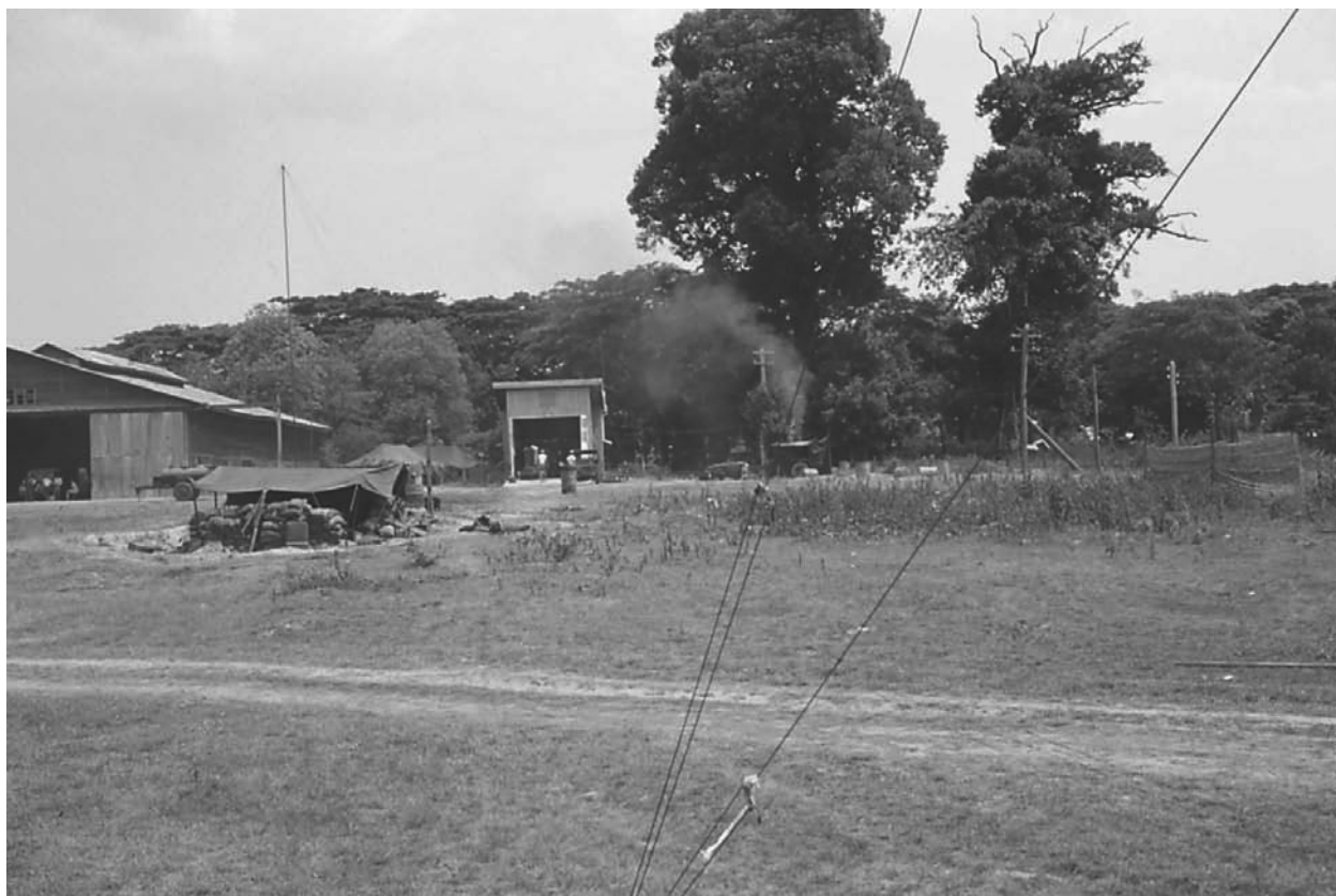
The communications center was established in a permanent structure outside of the main camp. The wires in the foreground held up a pole that provided elevation to the radio's antenna.
