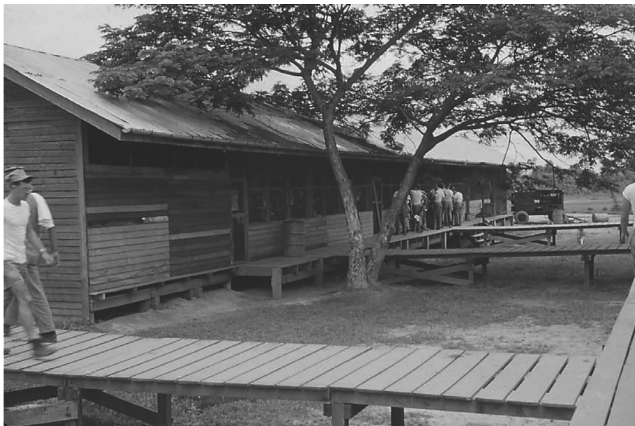
The squadron mess hall was located in one of the existing structures that had been rehabilitated by the engineers. Notice that it was built up off of the ground to prevent flooding during the monsoon season.
