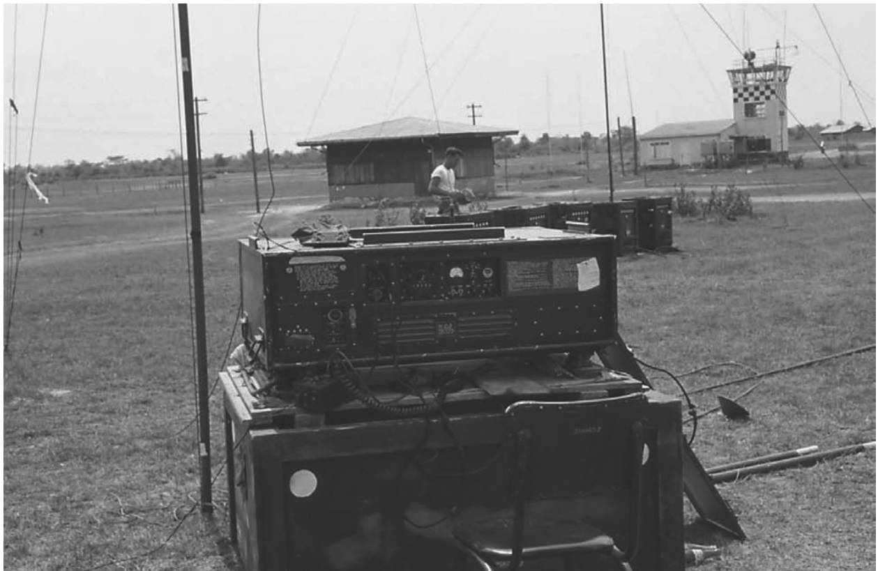
An AN/TRC-75 transmitter-receiver was set up outside of the communications center. The poles in the background supported the long-wire antennas that attached to the radio.
